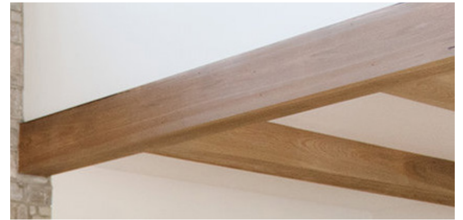
Beam detail: Add a beam over the entry to the dining space and run beams vertically in the room
