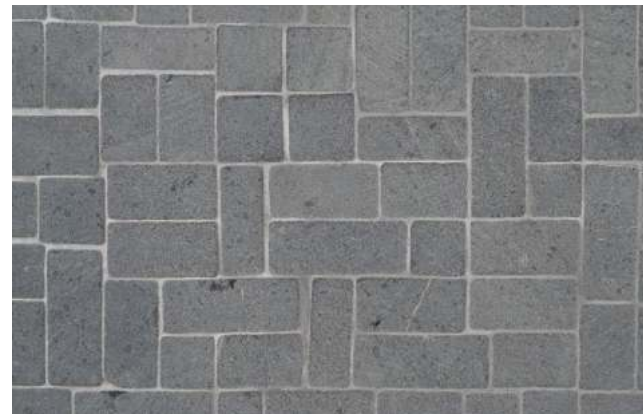
Floor tile throughout the bathroom and shower floor
