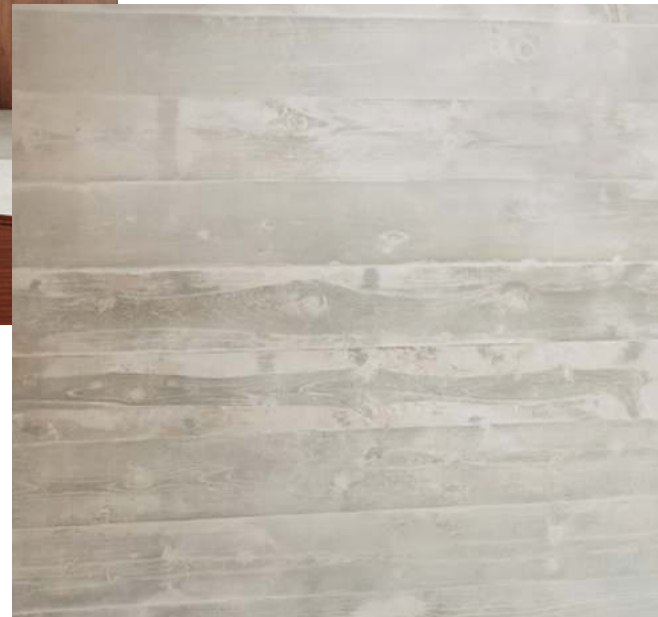
Board formed concrete
