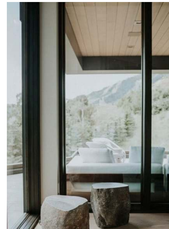
No door or window casings, just a drywall return for a modern
