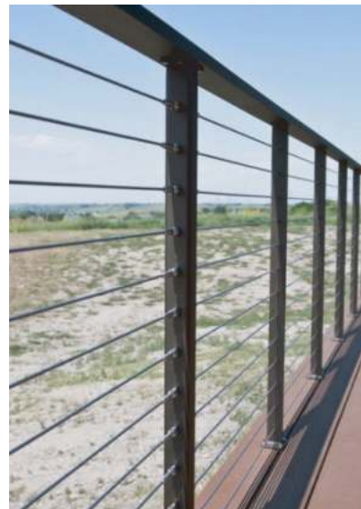
Railing: Modern metal posts and cables
